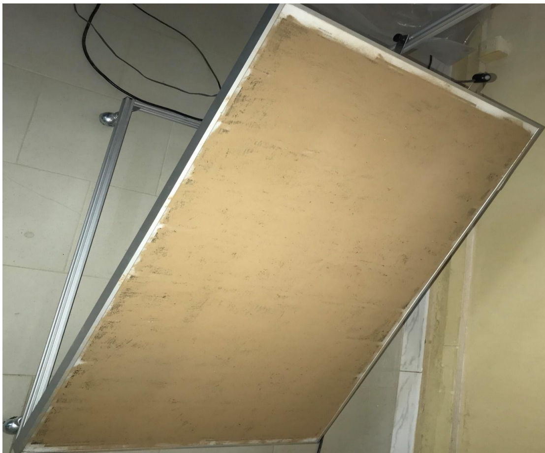
Figure 23. 6th year of deposit accumulation on the polycrystalline PV panel. Source: Author
